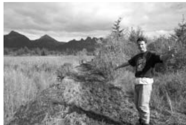
This is a section of the Alaganik Fisherman's Trail before trail construction showing severe damage to the muskeg.
